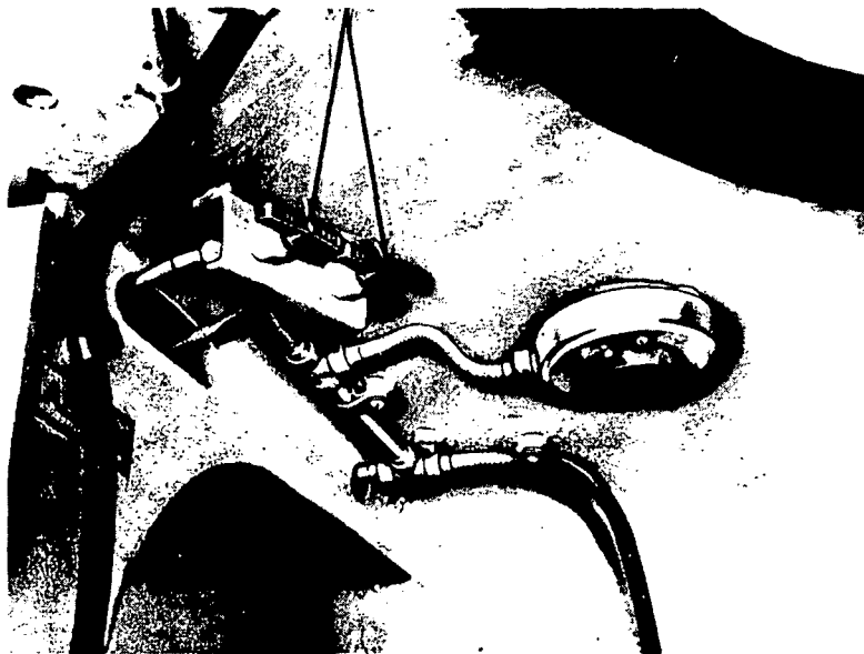
FIXED FIRE EXTINGUISHER CONTROL HANDLES
